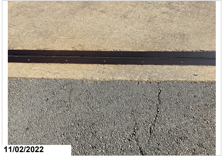
Abutment 1 has a few cracks in the top of the back wall.
