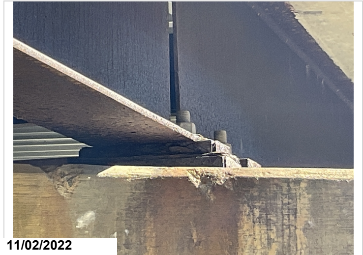
Bearings 1 and 5 have minor corrosion with flaking rust at bents 2 and 3.
