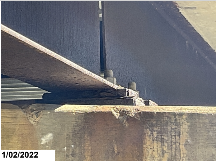
Bearings 1 and 5 have minor corrosion with flaking rust at bents 2 and 3.
