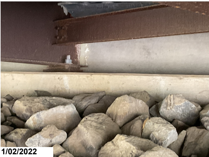
Abutment 1 has a few vertical cracks with efflorescence.
