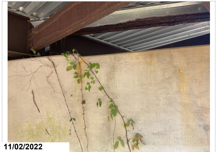
Bent 2 back side of cap has a vertical crack above column 2.
