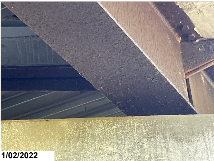
Girders 1 and 5 have minor corrosion on the bottom flange at bents 2 and 3.
