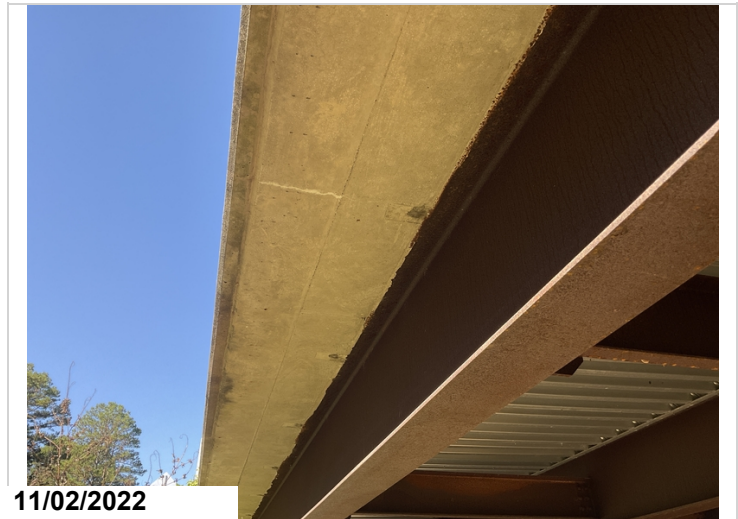
Soffit has cracks with efflorescence in the overhangs.
