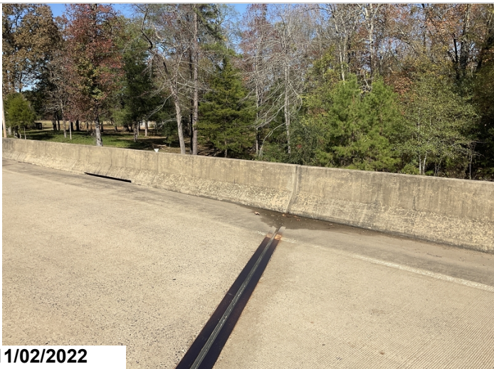
Concrete bridge rail has minor cracks that have been sealed.
