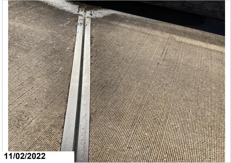
Deck has a few transverse cracks along the joints.
