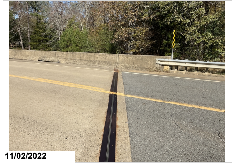
Typical condition of compression joints.
